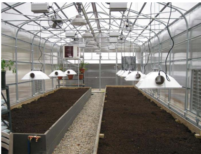
FIGURE 2-7: EXAMPLE OF LOW HANGING GROW LIGHTS
