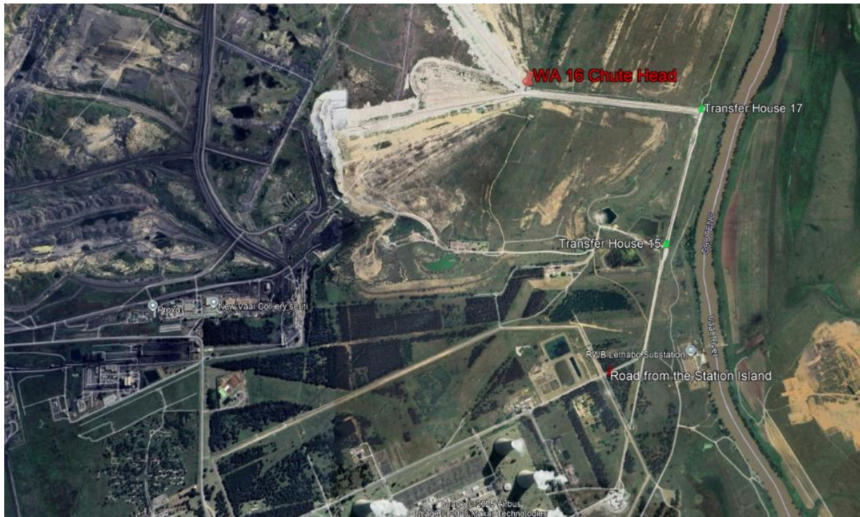
Figure 1: Location of the WA 16 chute
