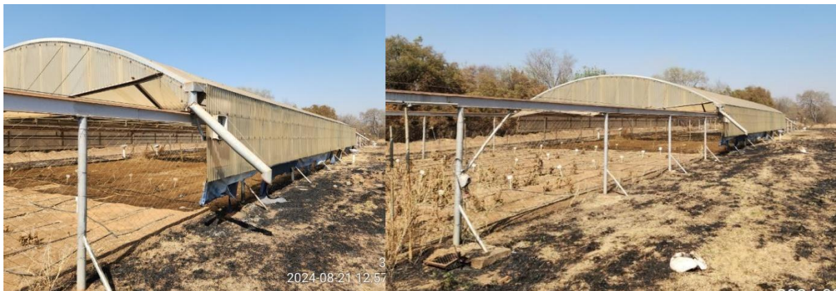
Photos of existing ARC structures
