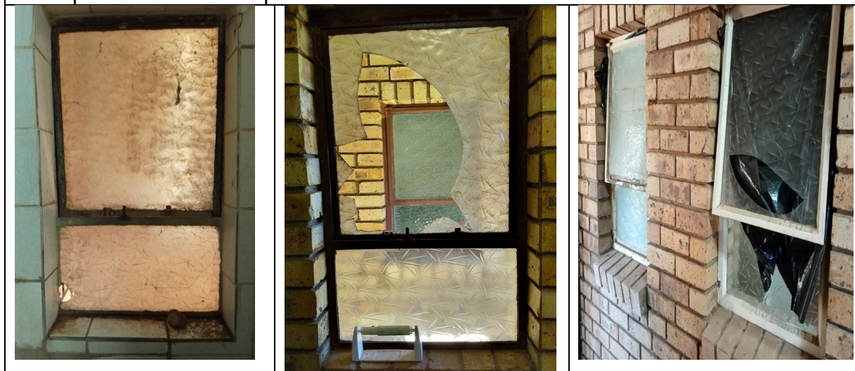
Examples of the work required on bathrooms and kitchen windows.
