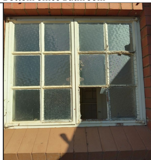
Bottom office Bathroom
