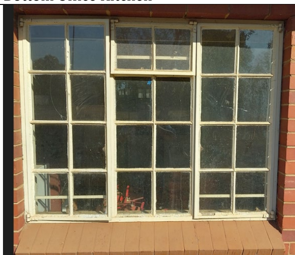
Bottom Office Kitchen
