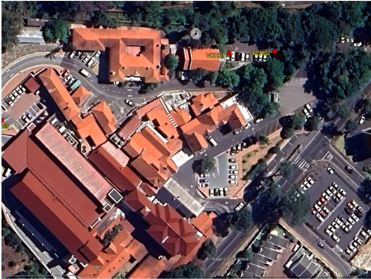
Figure 1: Location of the production boreholes at Victoria Hospital.
