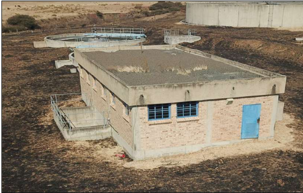
Figure 3: Arial View of Pump Station
