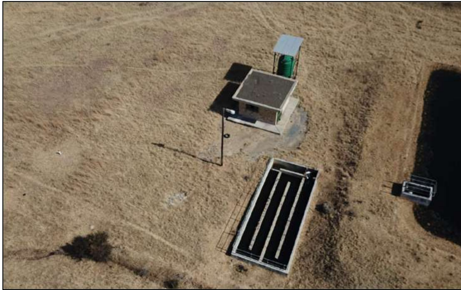
Figure 1: Arial View of Disinfection Facility
