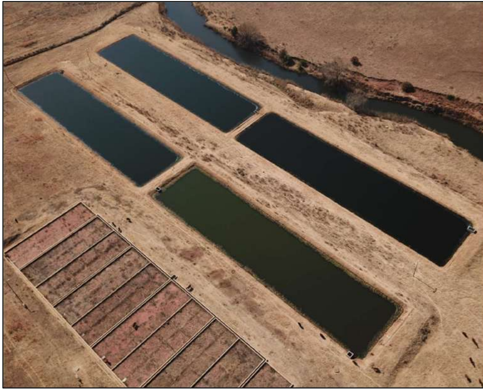
Figure 2: Aerial View of Oxidation Ponds
