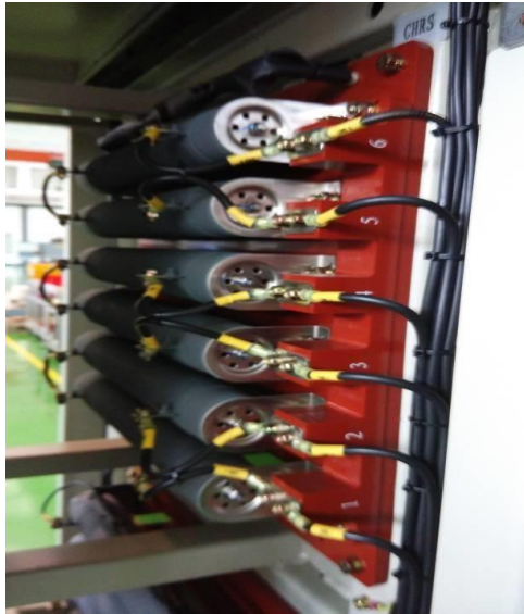
Figure 1: Charging Resistor
