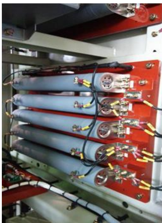
Figure 2: Discharge Resistor
