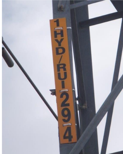
Figure 3: Line Tower Label
