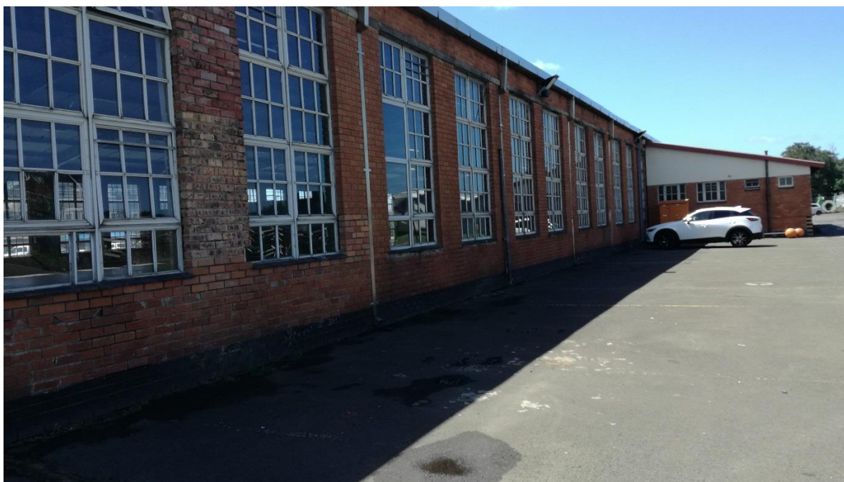
Figure 3: Rear View of Warehouse
