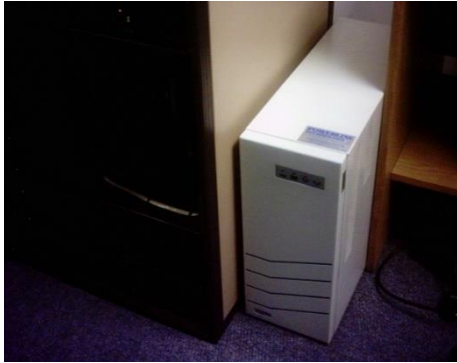
UPS in enclosed chassis mounted in MCC
