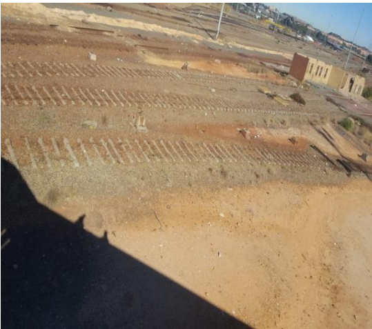
Fig 2.3: Vandalized staging yard
