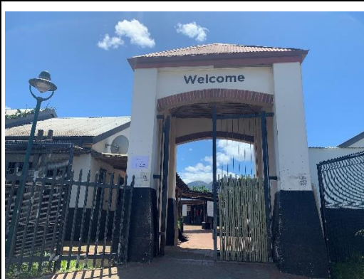
FIGURE 1.1: New paint to walls, steel gates and palisades
