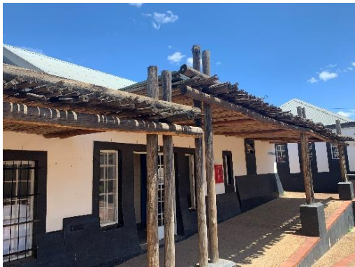
FIGURE 1.3: Removing and replacing gum poles and timber laths with steel structures and corrugated roof sheeting respectively
