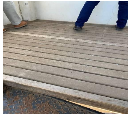
FIGURE 1.10: Sand, prepare and paint with new varnish to existing timber decking
