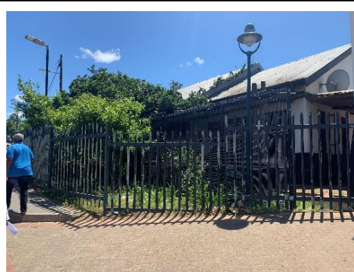
FIGURE 1.2: Removing of plants and replacing with new paving
