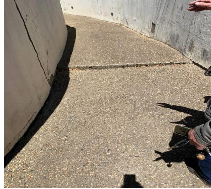
FIGURE 2.2: Demolish and rebuild existing concrete footpath to avoid hazardous trip
