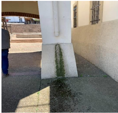
FIGURE 1.9: Install new missing uPVC gutters
