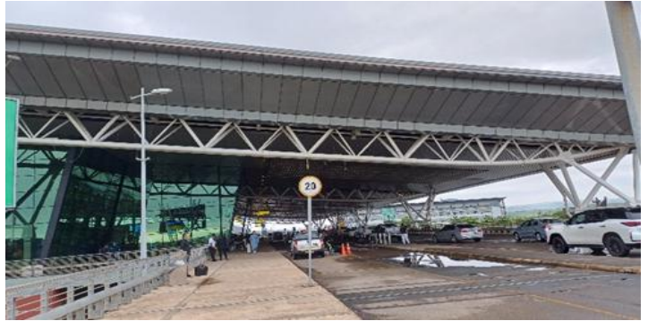
Drop Off Canopy
