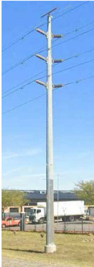
Photo 1. Typical Intermediate Structure
