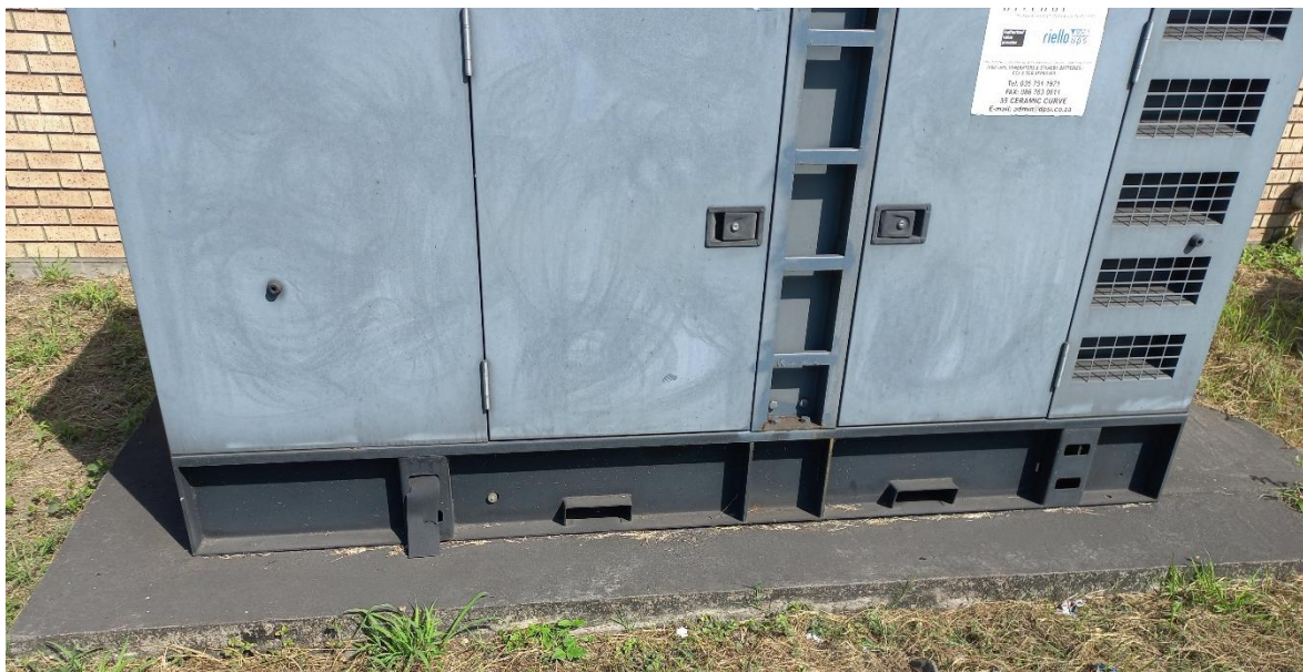
Figure 2: Similar Concrete Plinth for Berthing Generator.
