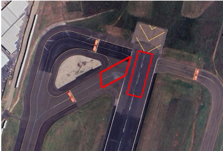
Figure 1: Quebec Taxiway and 21R Runway Threshold
