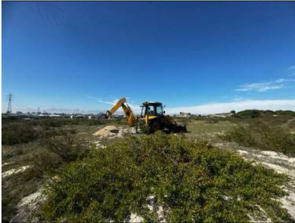
General View of Site
