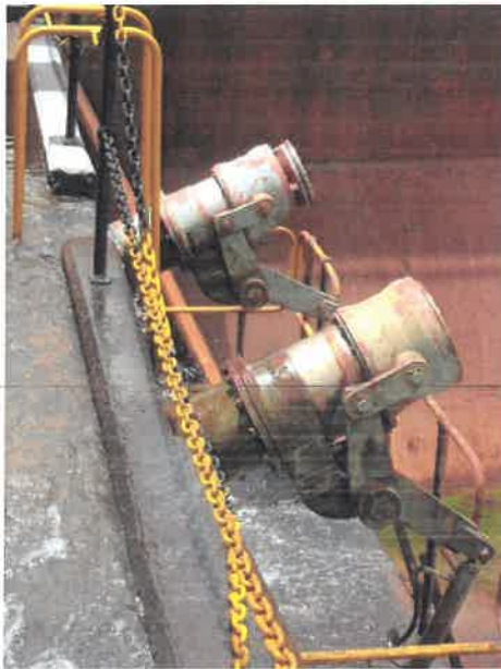
Sleeve valve installation
