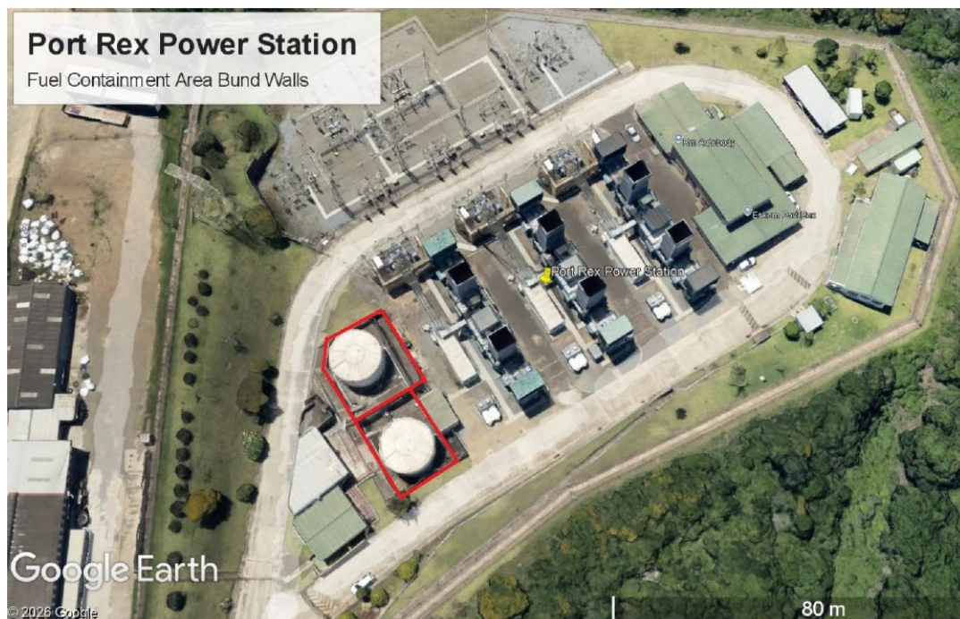
Figure 1: Fuel containment area bund walls at Port Rex Power Station*(highlighted in red)
