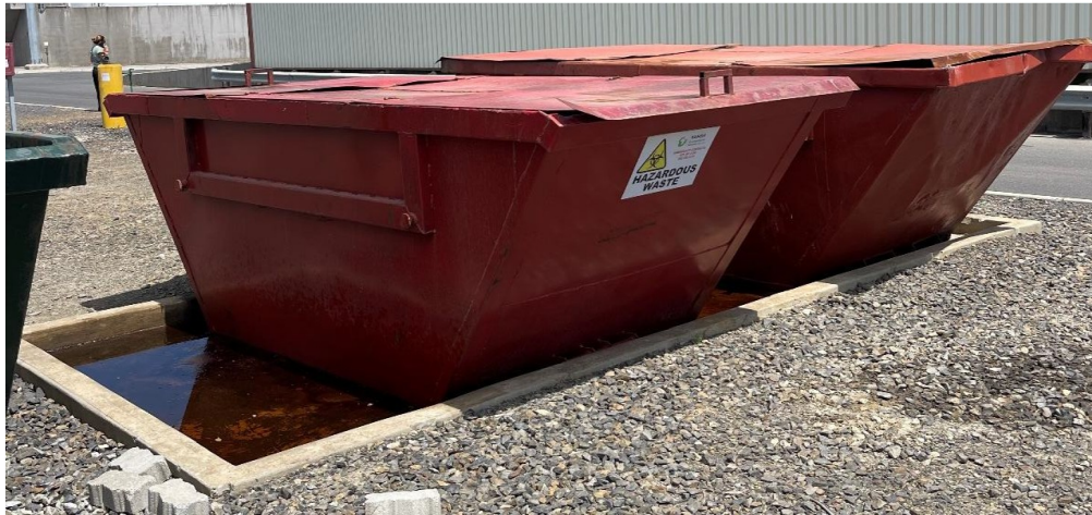
Figure 2: Example of existing waste Skip Storage
