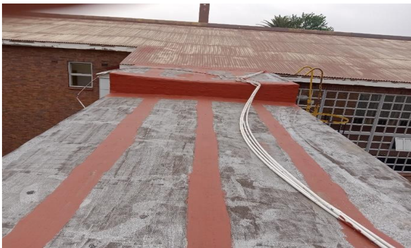
Figure 3: Main Administration roof slab
