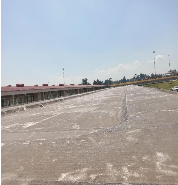
Figure 2: No.3 Mcc and blow house
