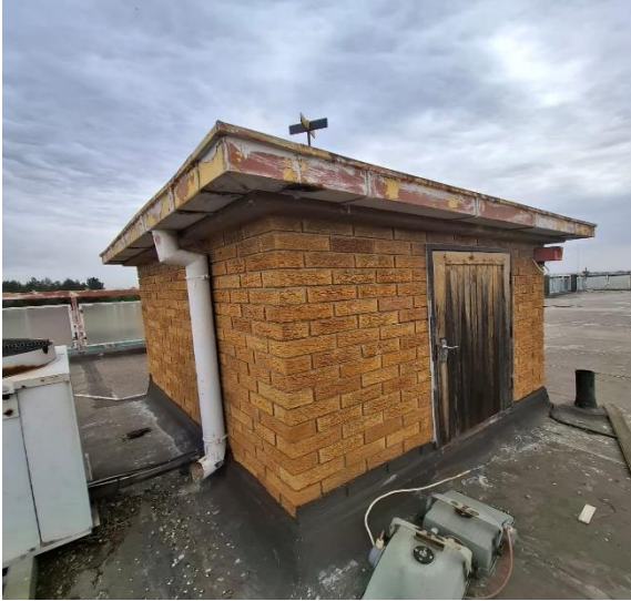
Figure 6: No. 3 Roof Access tower
