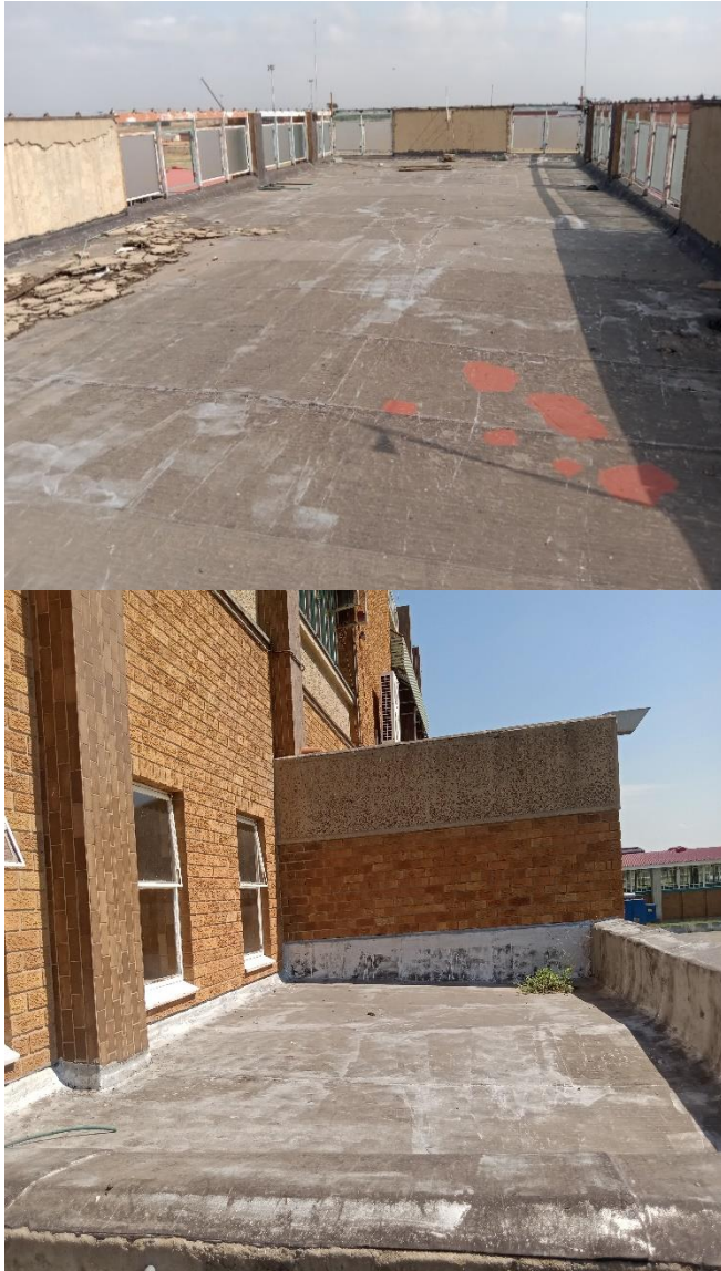
Figure 1:No. 3 Control roof slab
