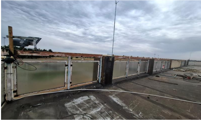
Figure 5: Balustrade to be painted.
