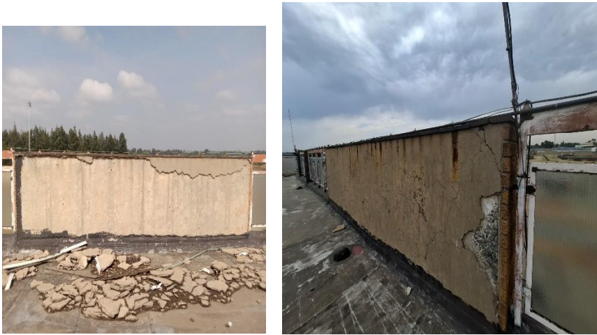
Figure 4: No3 control boundary walls
