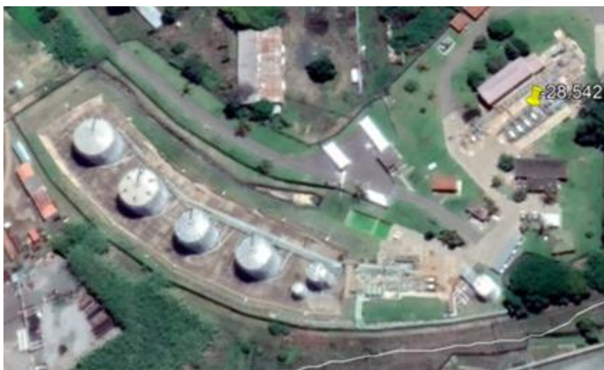
Figure 2. Ariel view of the Ladysmith depot
