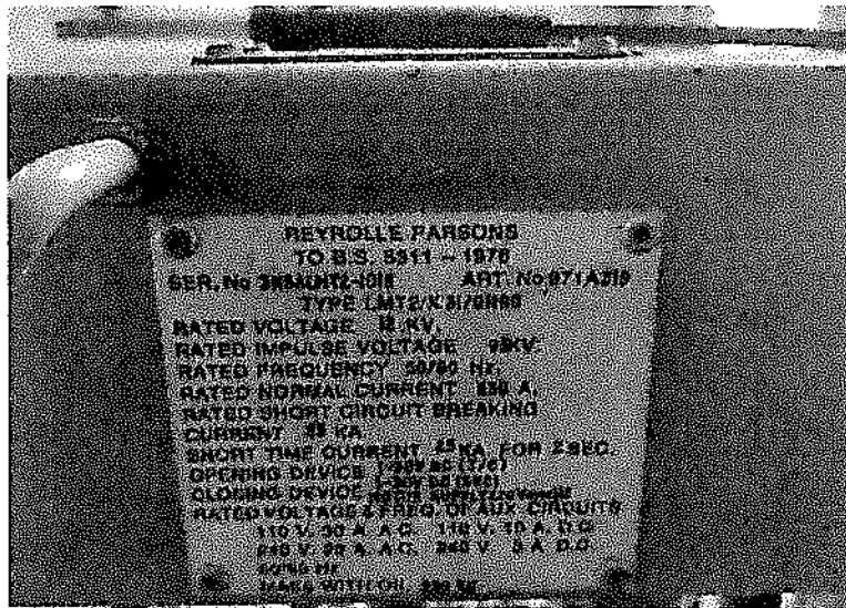
Image B.2.4 - Main isolating contactors of OCB
