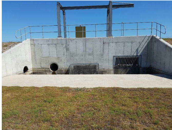
Figure 8 - Close-up of the inlet and outlet at Foxtrot 5 pond.
