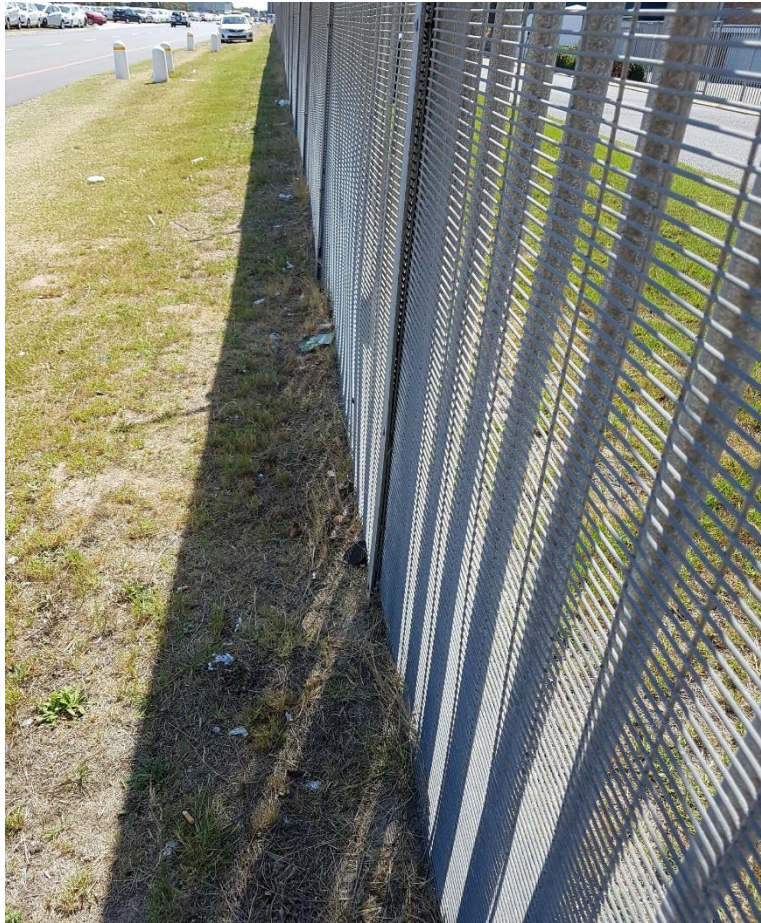
Figure 5 – Close-up of the fence on the Southern Access Routes that must be sprayed with a non-selective herbicide.
