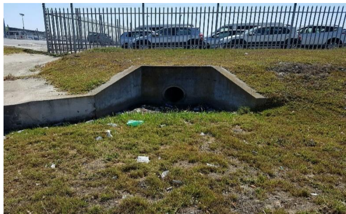
Figure 6 - Inlet and outlet of the Beechcraft Road Pond that must be kept free flowing.
