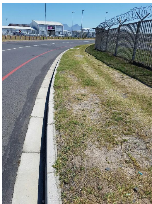
Figure 4 - Southern Access routes showing kerb and fence that must be maintained.
