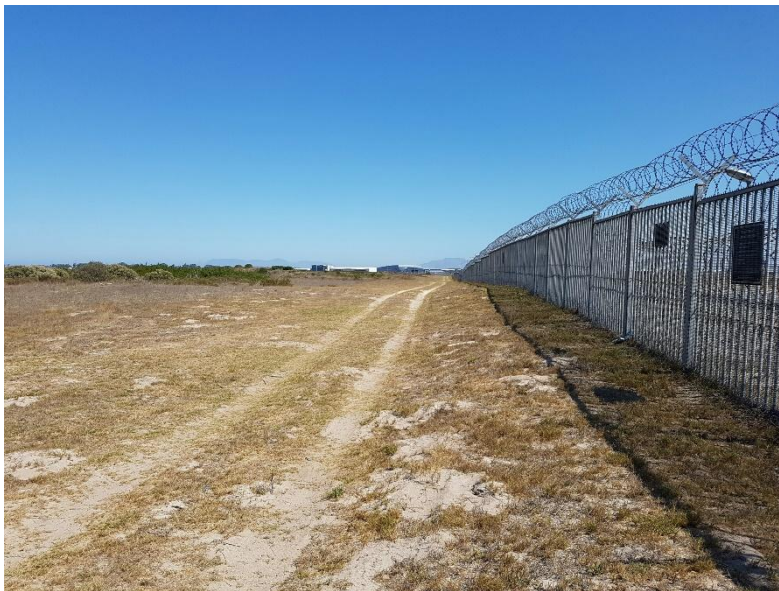
Figure 2 - 15 metre Fire break on the outside of the fence.
