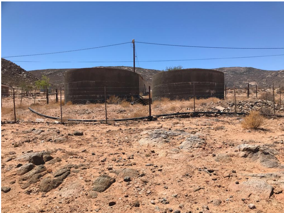
Figure 3: Showing water tanks.
