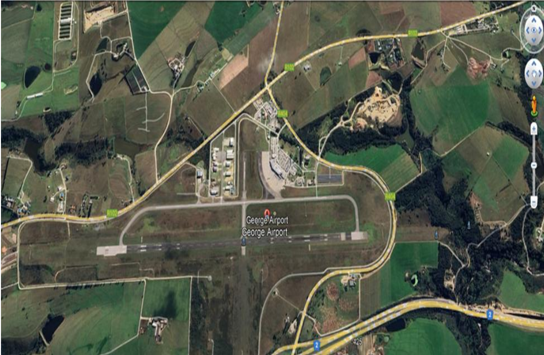
Figure C4.1: GRJ Aerial View Image
