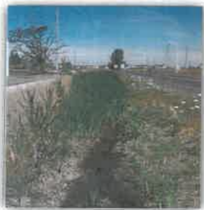
Typical application of a deflection berm to avoid erosion of a pipeline route
