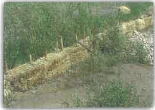
Figure 3 Hay bales used for silt retardation
