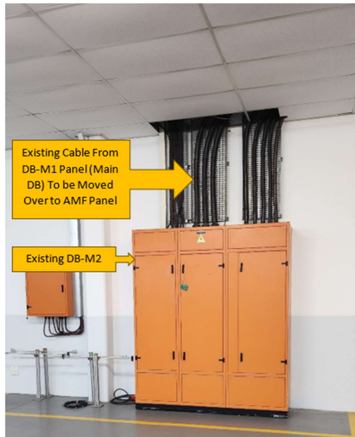
Figure 5 Proposed Cables That Require Relocation
