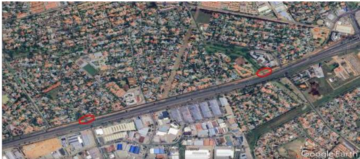
Aerial Map of the project site and areas that requires Erosion Control Structures Corrections.
