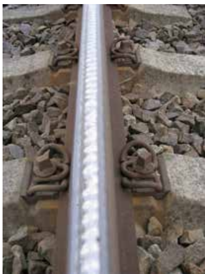
Figure 9 — Short pitch corrugation
