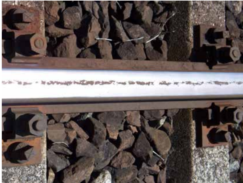
Figure 5 — Spalling
