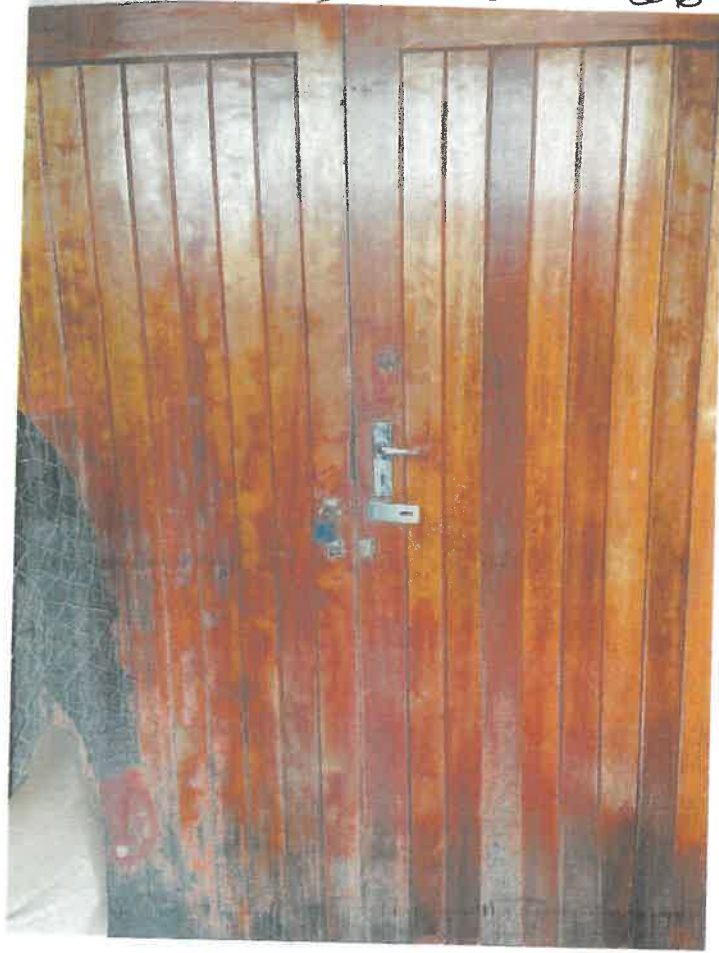
Main door room 26
