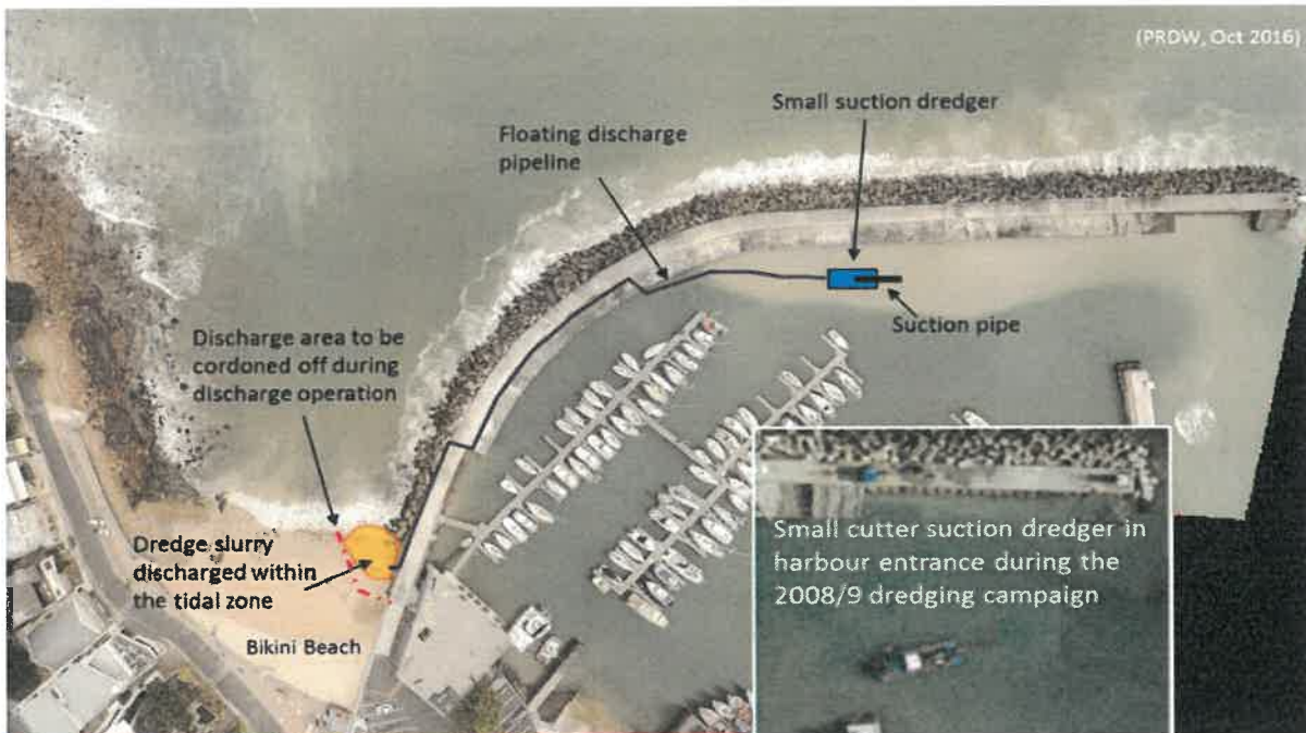
Figure 1: Indicative maintenance dredging operation and sand discharge.
