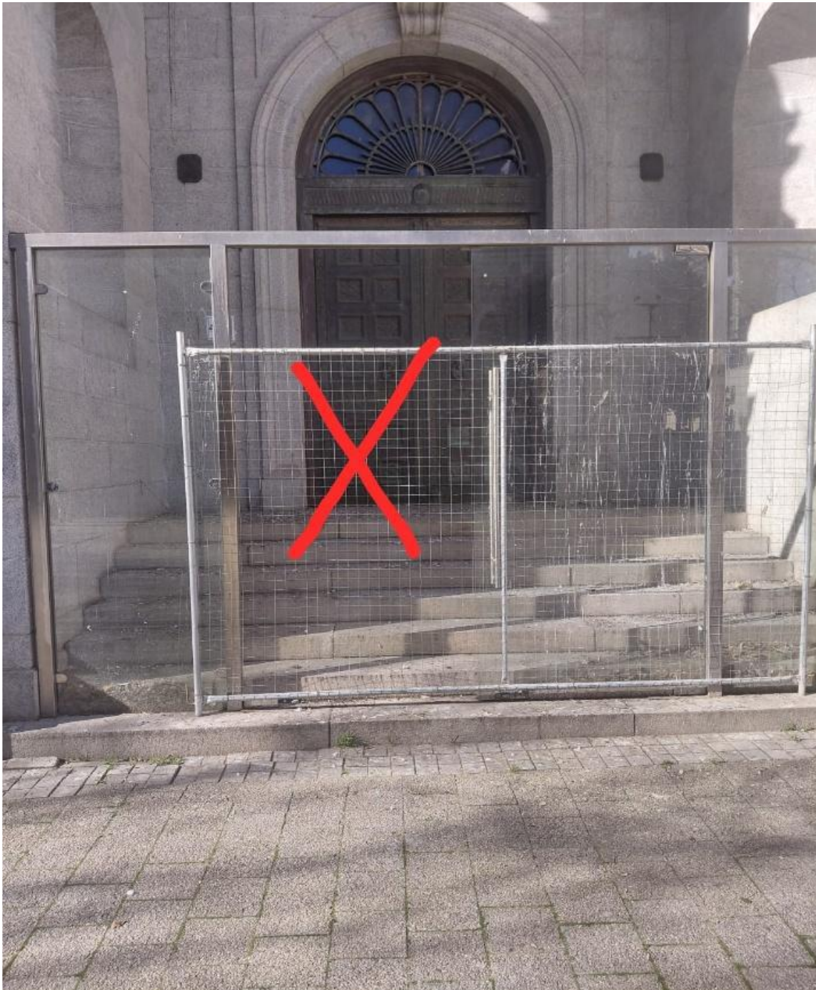
Figure 7. Install three large frameless glass panes between pillars near staircase
