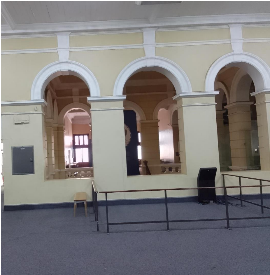
Figure 5. Supply, deliver and install three (3) 6 mm clear toughened safety glass infill panels
