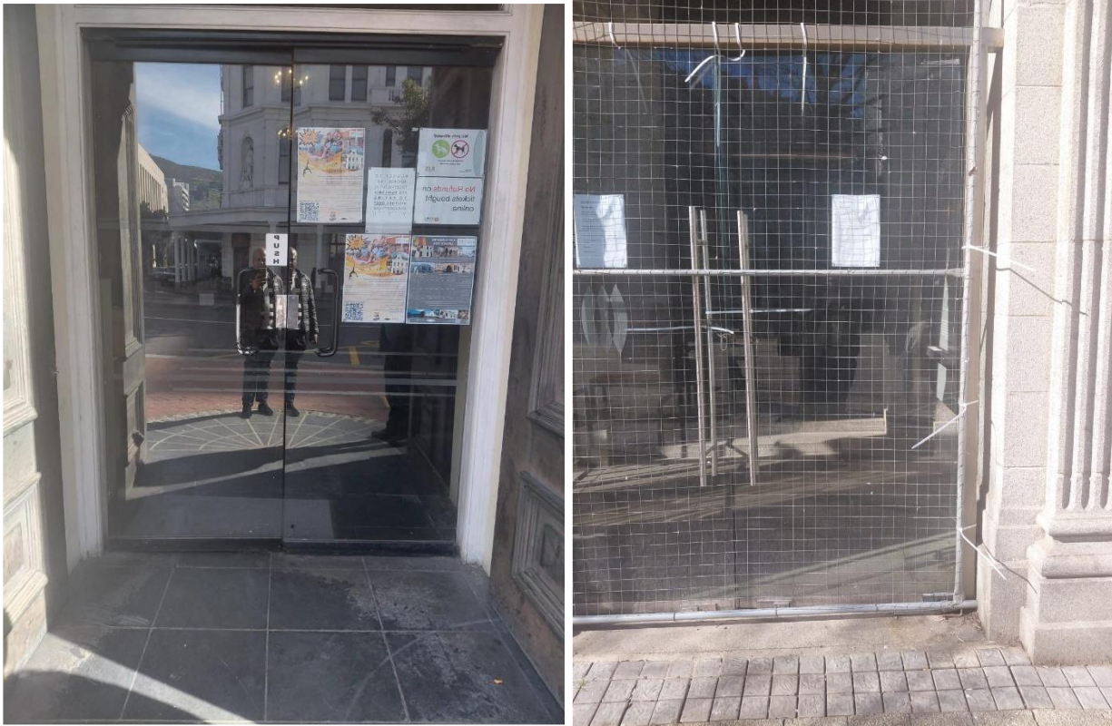
Figure 6. Install three large frameless glass panes between pillars near staircase
