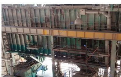
Bin 1 top panel replacement
