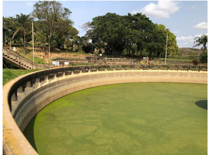
Clarifier (2) Photo 10-Water in Tank
