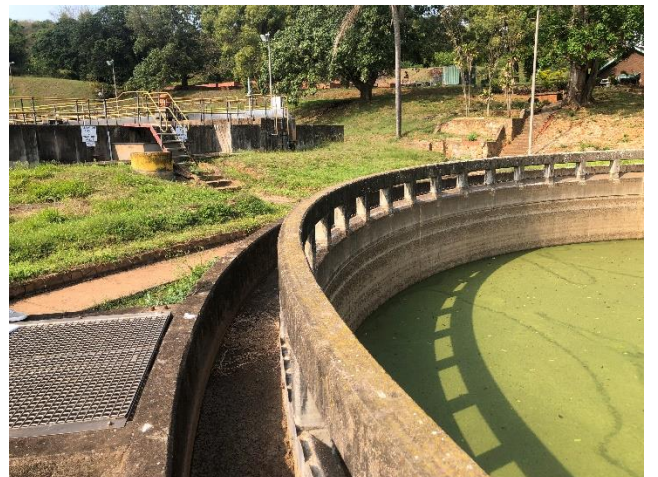
Clarifier (1) Photo 02-Sludge Deposition
