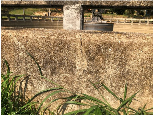
Clarifier (1) Photo 04-Outer wall cracks (0.2-0.3mm)
