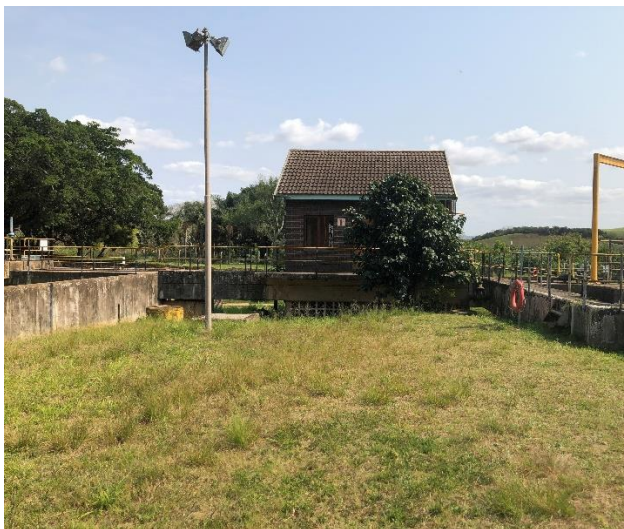
Screw Pump Room Photo 11-Elevation
