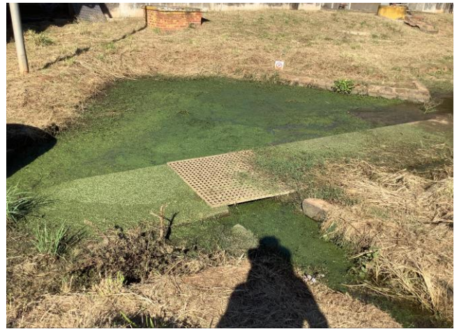
Clarifier (1) Photo 01-Sewage spill
