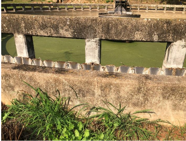
Clarifier (1) Photo 04-Outer wall cracks (0.2-0.3mm)
