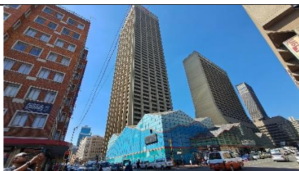
Office Tower - corner Main and Von Wielligh street
