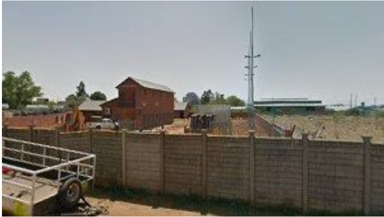
Figure 1 – Street View of Muncip Substation
