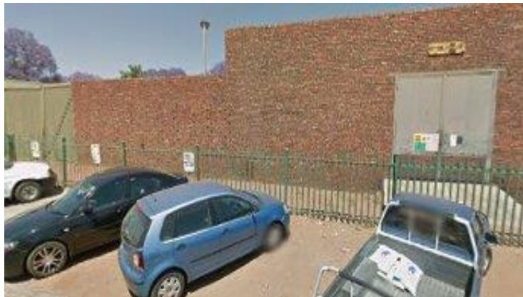
Figure 3 – Street View of Park Substation
