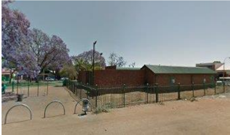
Figure 4 – Street View of Park Substation
