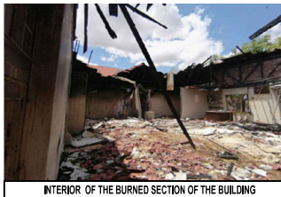
INTERIOR OF THE BURNED SECTION OF THE BUILDING
