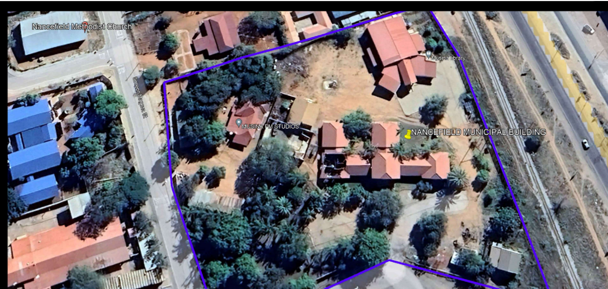
PROJECT SITE - MUNICIPAL BUILDING TO BE REFURBISHED
