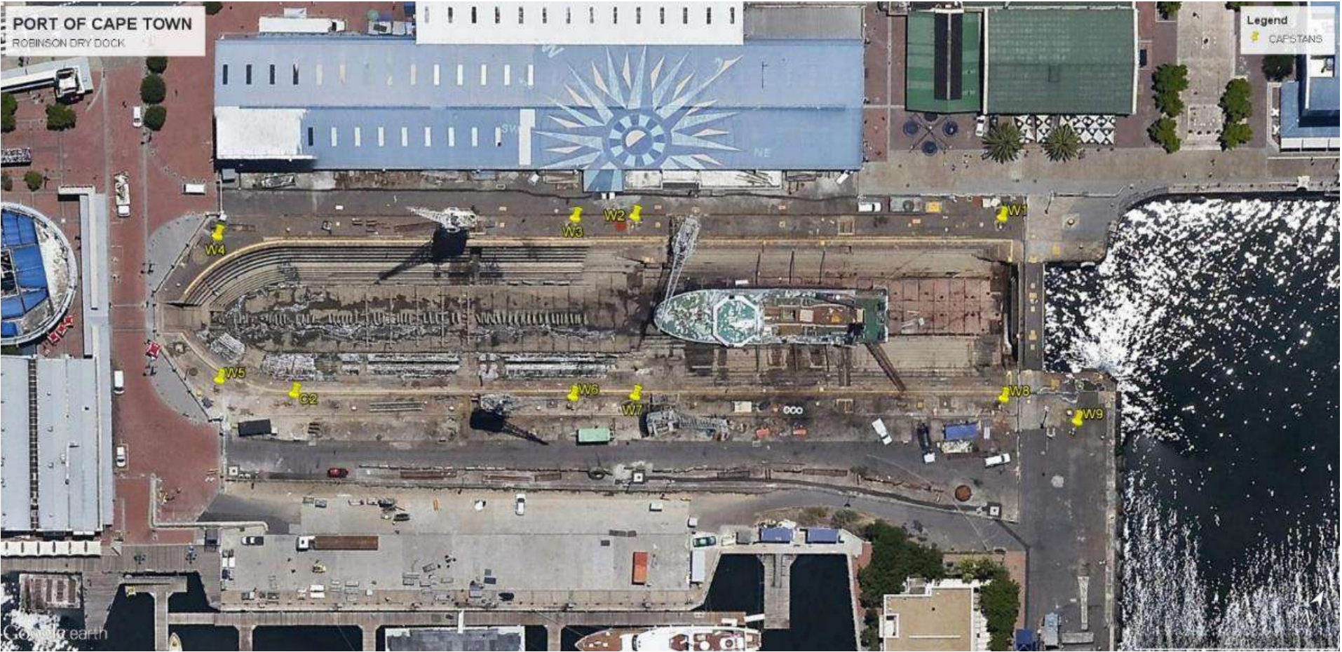
Figure 3: RDD Capstans Port of Cape Town
