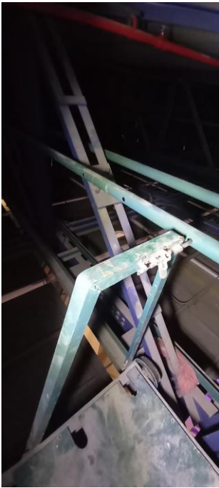
Figure 3 Braking pins on trolleys.
