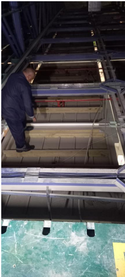
Figure 4 Safety board to be installed for safer access to winches.
