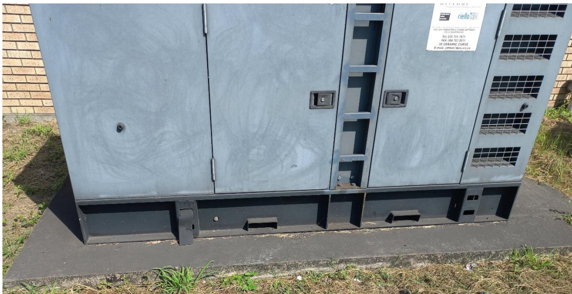
Figure 2: Similar Concrete Plinth for Berthing Generator.
