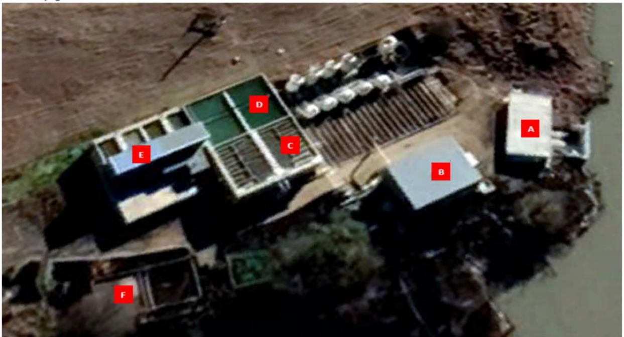
Figure 1: AMERSFOORT WATER TREATMENT PLANT
