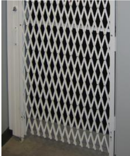
Figure 2: Example of the trellis door/gate
