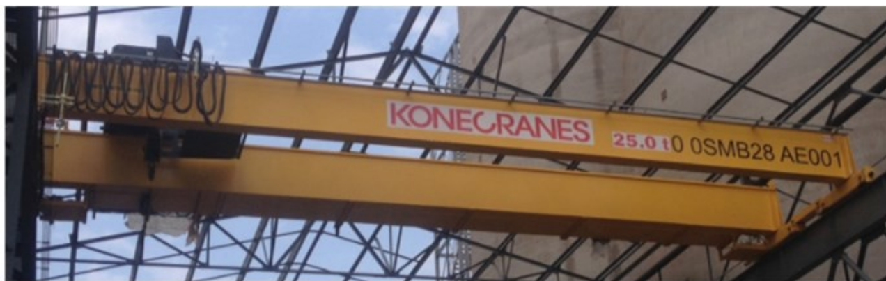
Figure 34: Crane and crawl beam stencilling
