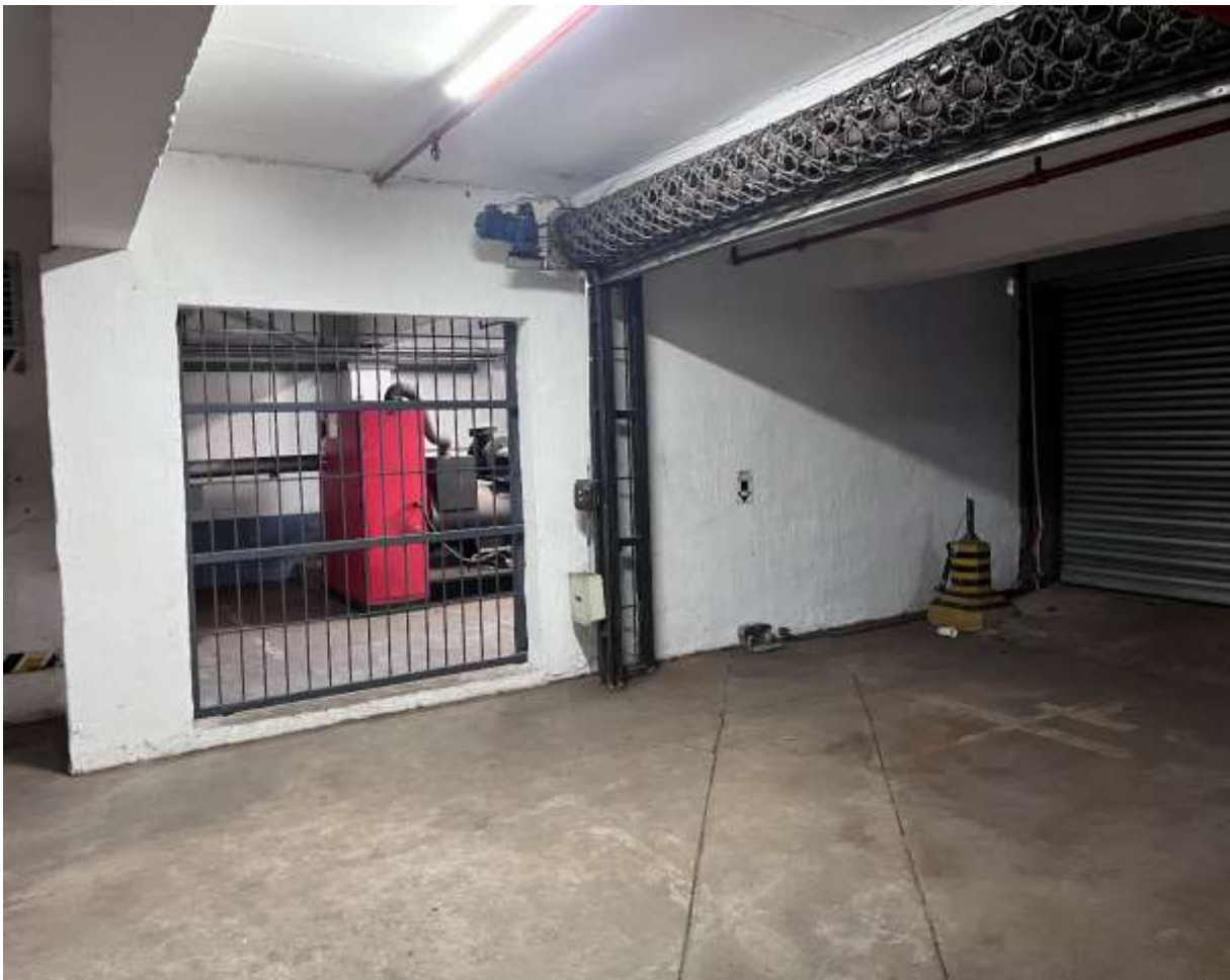
Generator wall to be removed/ demolished for access
