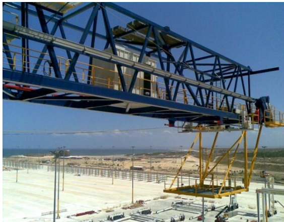
Figure 24: Back of STS
