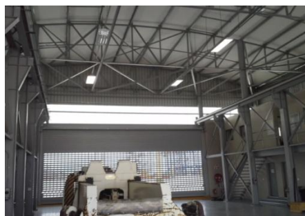
Figure 44: RTG workshop inside (340 m2)
