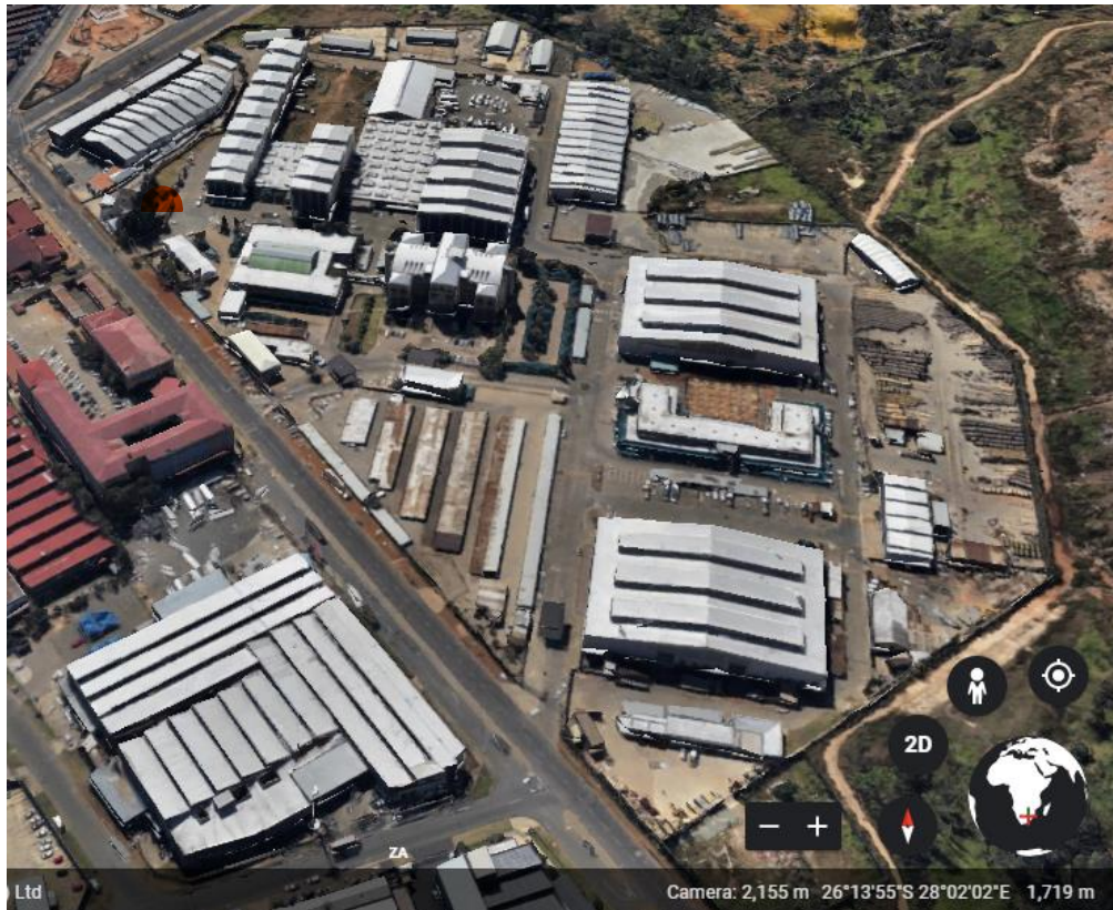
Figure 1 : Facility aerial view
