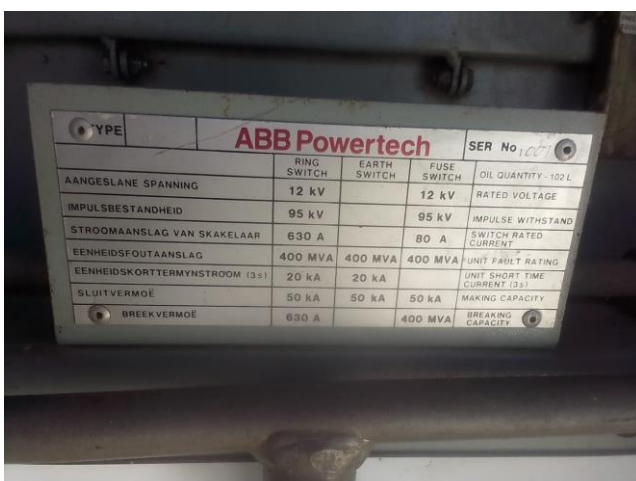
Figure 3 – Air-BP Minisub Circuit Breaker
