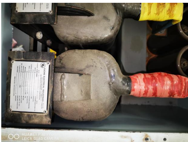
Figure 2 - 11kV CT's
