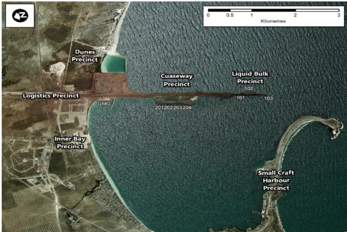
Figure 7: Port of Saldanha Aerial View
