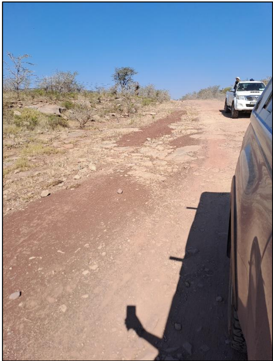
Plate 3 (Left): Deeper transported finer grained soils at TP1 and TP2. Plate 4 (Right): Sporadic rock at surface between TP5 and TP6. Note TP6 with weathered mudstone from surface throughout cut extent.
