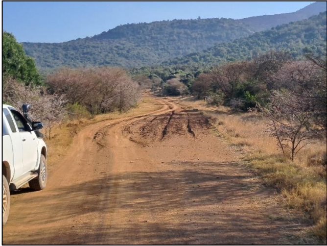
Plate 1 (Left): Worn and entrenched tracks through existing road layers underlain by fine grained materials between TP1 and TP2. Plate 2 (Right): Surface pooling on fine grained subgrade at TP1.
