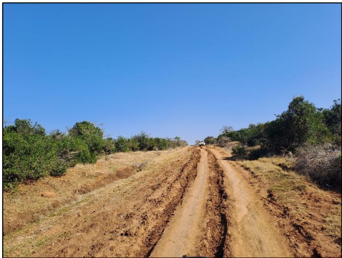
Plate 1 (Left): Worn and entrenched tracks through existing road layers underlain by fine grained materials between TP1 and TP2. Plate 2 (Right): Surface pooling on fine grained subgrade at TP1.
