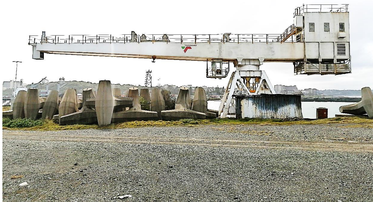
Figure 2: Breakwater Crane post refurbishment in 2019/20
